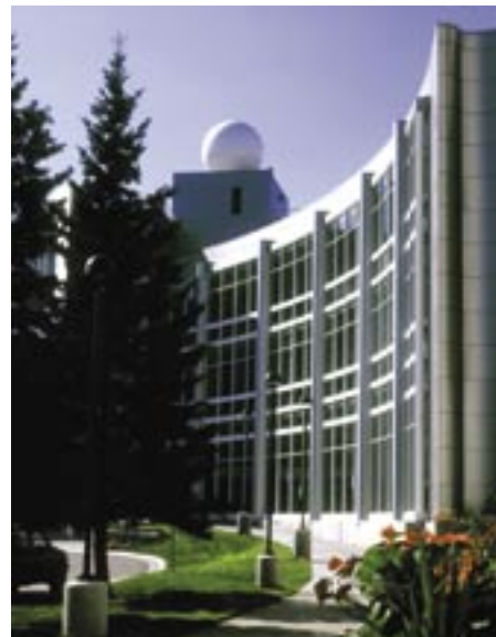
The antenna will use a Moderate Resolution Imaging Spectroradiometer that will enable scientists from the University of Alaska to view Alaska from above. Photos of the antenna were taken by Jeff Pederson of the Geophysical Institute Digital Design Center.
