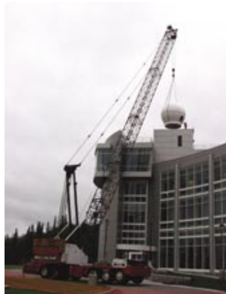
In August 2001, contractors and Geophysical Institute researchers assembled a new antenna and installed it on top of the International Arctic Research Center.
