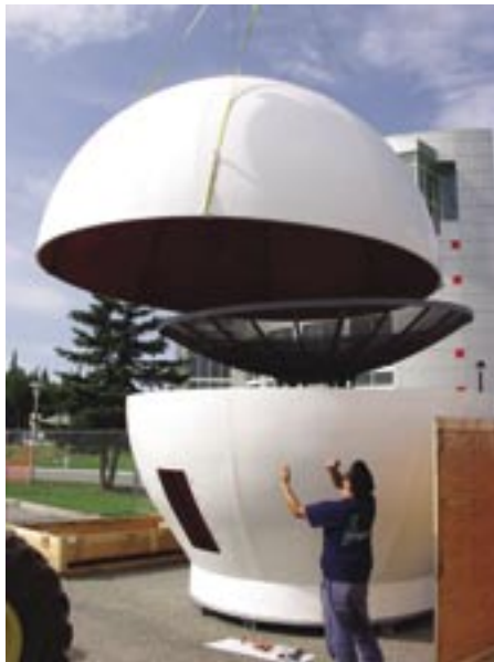
In August 2001, contractors and Geophysical Institute researchers assembled a new antenna and installed it on top of the International Arctic Research Center.
