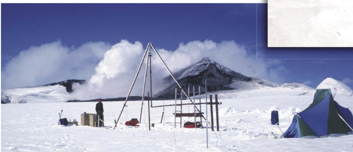
MONITOR—Senior Project Engineer Steve Estes installs and monitors seismic equipment on Mt. Wrangell.
