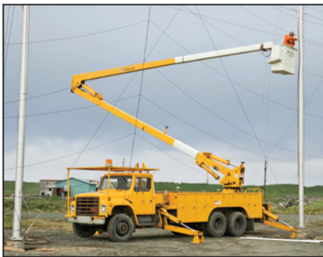
INSTALLATION —Kevin Sterne of Virginia Tech connects antenna wires to one of the 55-foot support poles at the Adak site.
