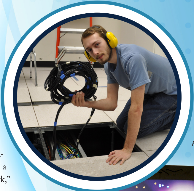
Tim Slauson, ARSC research project assistant, runs cables under the Butrovich Machine Room floors. Photo by Azara Mohammadi.
