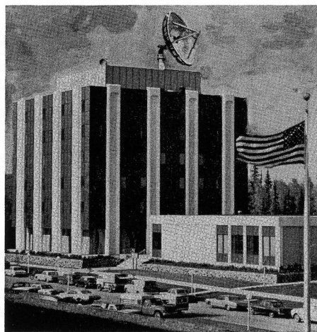
Artist's concept of the new radar antenna to be installed on the roof of the Elvey Building.
