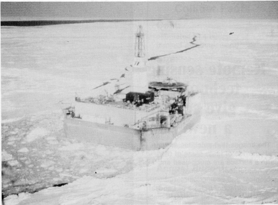
Gulf Canada's Malikpak, an offshore oil drilling structure, surrounded by annual ice, 1985. (Photo courtesy of K.R. Croasdale.)
