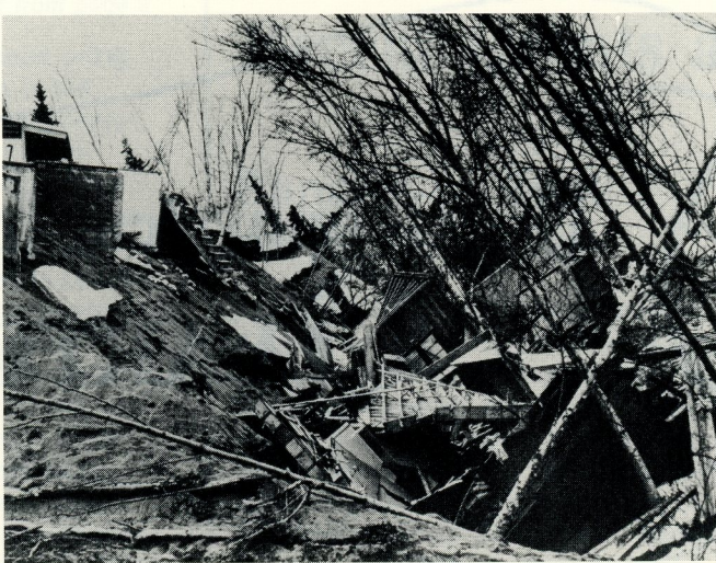
A home destroyed near Anchorage during the 1964 earthquake. Seismology research such as that done at the Geophysical Institute is essential in predicting where earthquakes will occur. (J. Townsend photo, College Observatory collection.)
