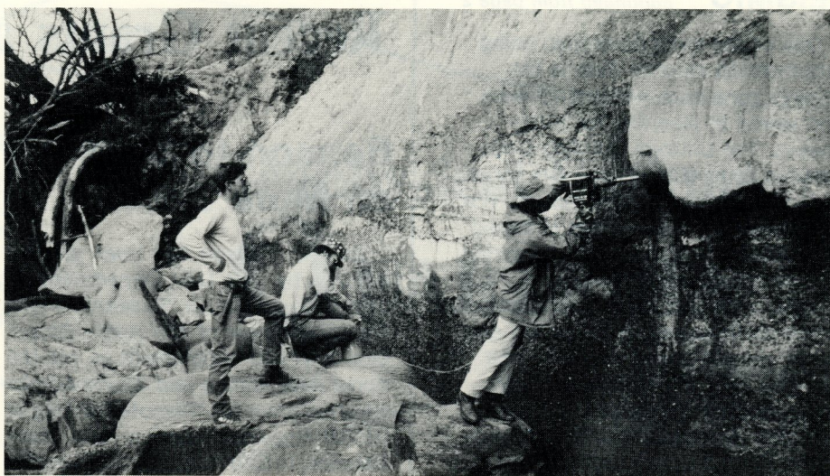
Geophysical Institute researchers are shown drilling a rock core sample in Kachemak Bay. The direction of the magnetic field in bedrock helps define the "terranes," and thus aids in locating gas, oil, or mineral deposits. (D. Stone photo.)
