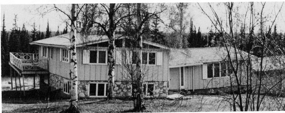
Damaged by the settling of thawing permafrost under the foundation, this house had to be abandoned while it was still fairly new.
