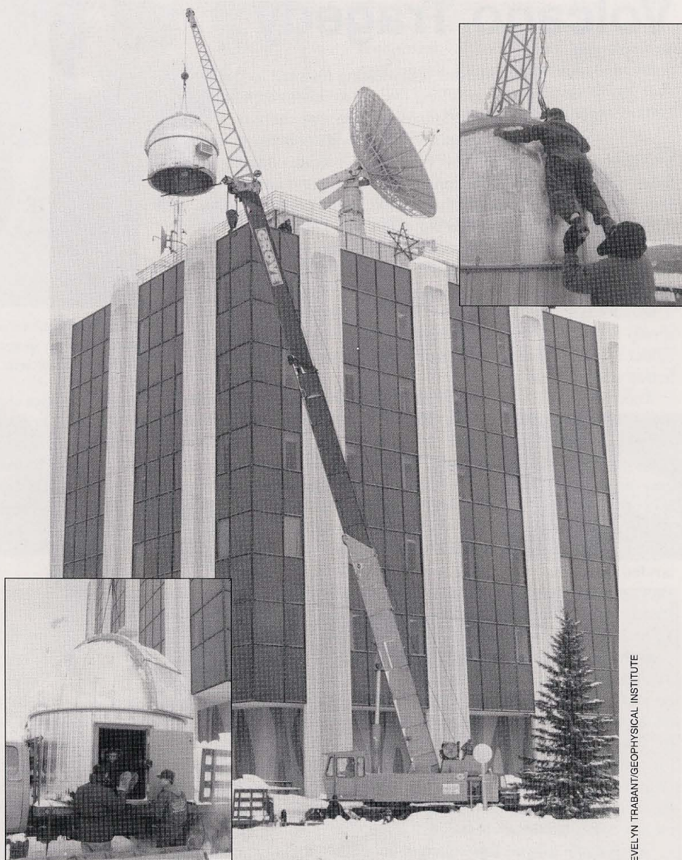
On Top of It —Research Assistant Jim Slusser confers with crane operators, lower left, before the dome shelter for the Dobson instrument is hoisted to the top of the institute. Once on the roof, more than 40 graduate students carried the dome into place. Ray Ward removes the crane cables, upper right.
